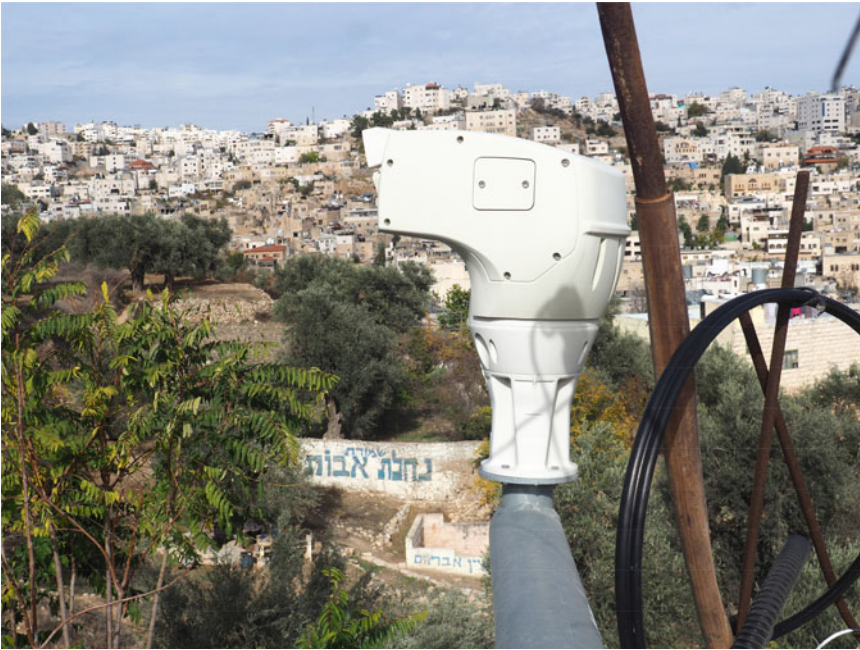
Figure 2. Military surveillance camera installed on the roof of a private Palestinian home in the Old City, with the remainder of Hebron in the background. Photo by author.
