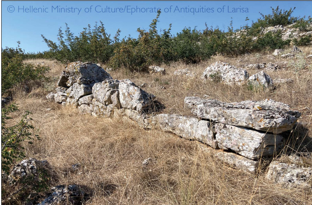
Figure 8. Fortification wall on the hill of Chtouri (©Hellenic Ministry of Culture and the Hellenic Organization for the Development of Cultural Resources; photograph by author).
