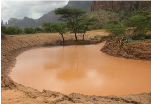
Fig. 6.26 Percolation pond (left) captures runoff from the scarp at Koraro. The water is allowed to percolate into the subsoil, and is pumped from shallow wells lower in the landscape where farmers have their fields (right).
