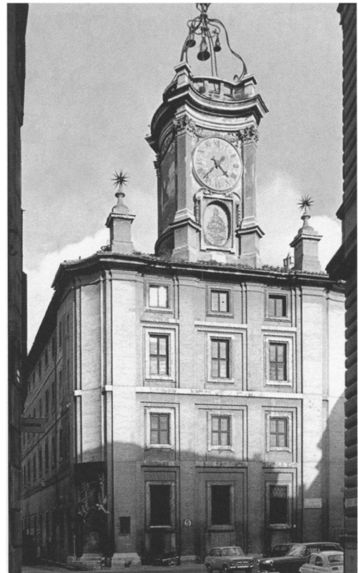
Fig. 22. North-west corner of the Oratory House, with the clock tower built in 1647–50
