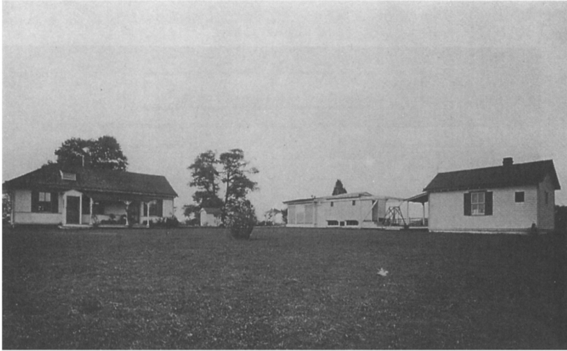
Figure 6. General view of grounds of Gaithersburg ILS station. The site was named a national historic landmark in 1990. From Ross (1915).
