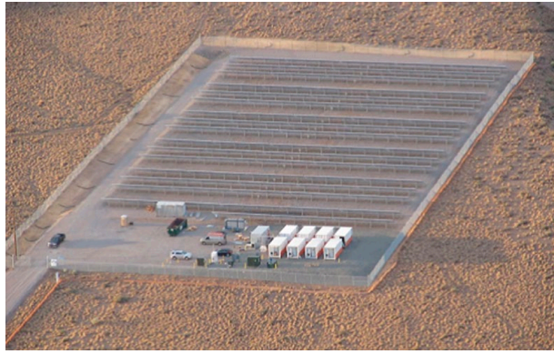
Figure 2. Aerial view of the Prosperity Electricity Storage Project in New Mexico, USA 56 (reprinted with permission).
