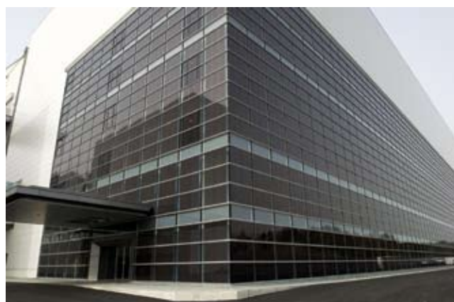
Figure 2. Thin-film “see-through” solar cells covering the windows of an office building.
