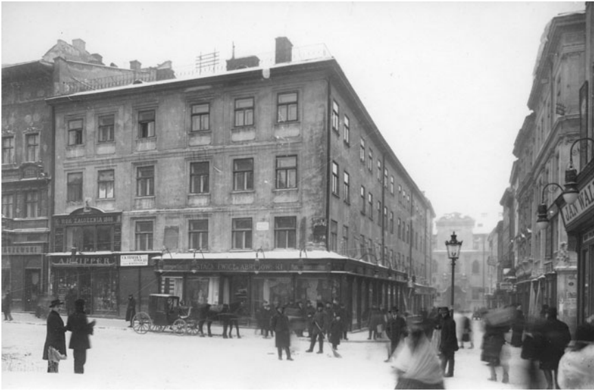
Figure 3. The old Zipper House before demolition in 1912, as seen from the Main Square. Source: Centre of Urban History of East Central Europe, ID no. 3548.
