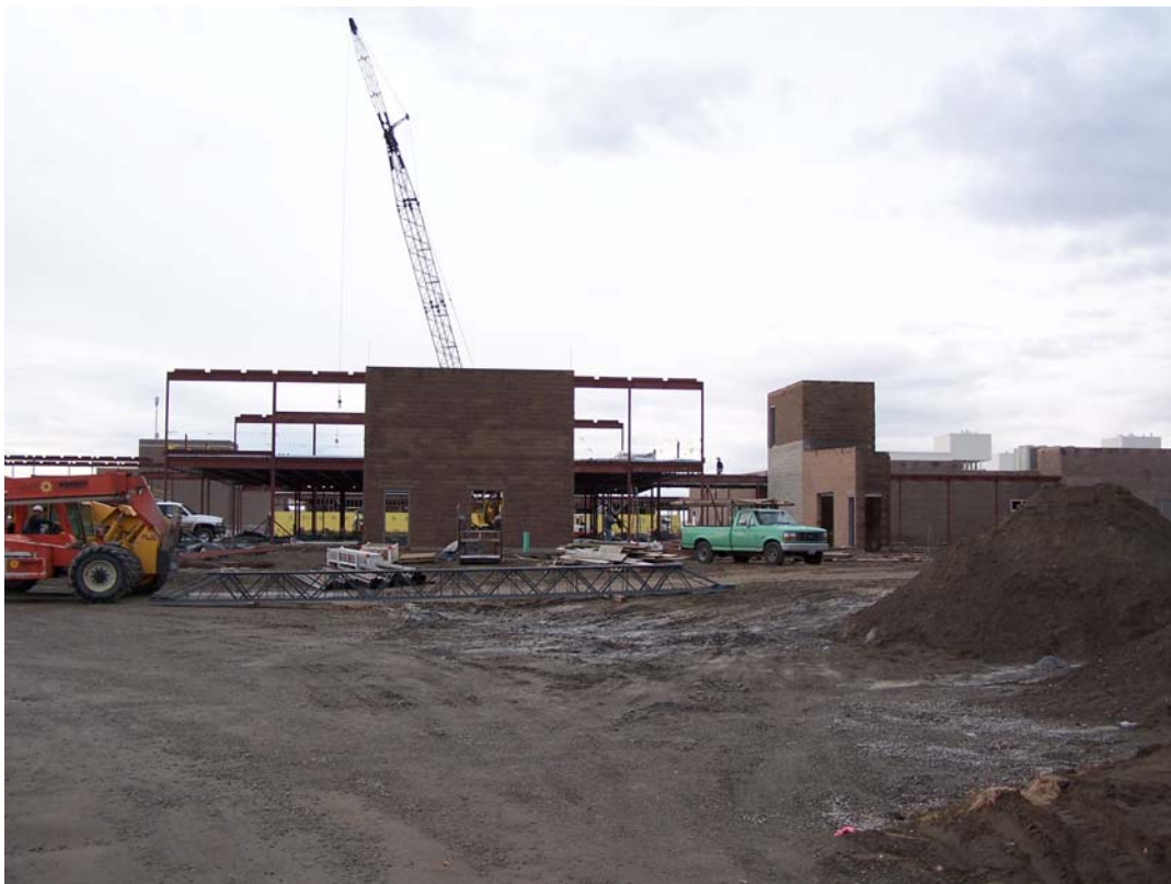
Under construction at the campus
