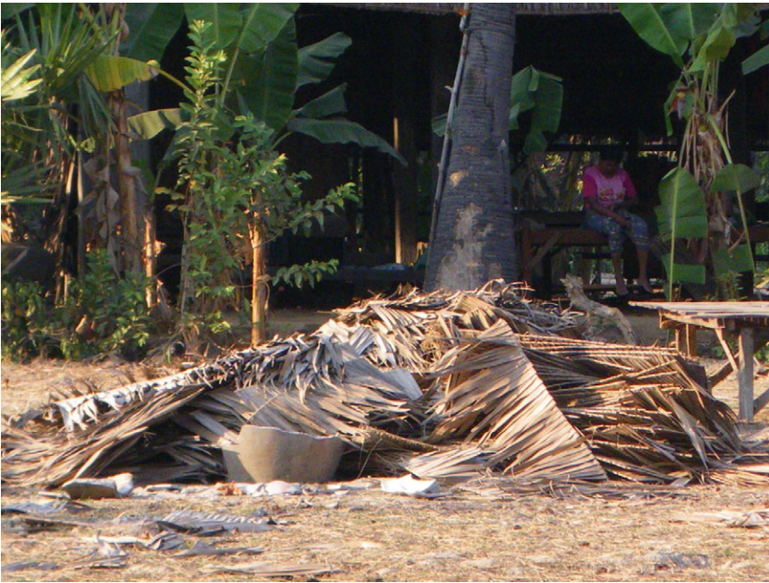
Figure 6. A shack demolished by the DPOC in 2010 (courtesy of the author).
