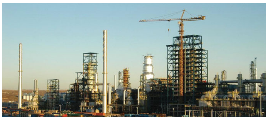
China's coal producer, the Shenhua Group, owns the world's largest facility to convert coal into liquid fuels using direct liquefaction technology. The plant, located in Inner Mongolia, started operations in 2009 and produces 24,000 barrels of diesel and gasoline a day. Credit: West Virginia University.
