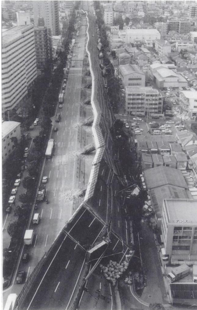
Figure 1. A ruined motorway (©Yomiuri Newspaper Company)
