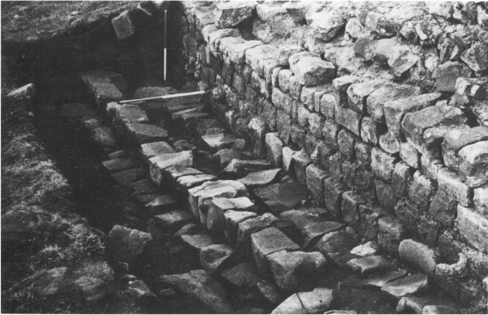
A. Hadrian's Wall, High Shield Crag: Broad foundation, Narrow foundation and later reconstructed Narrow Wall (p. 280).
