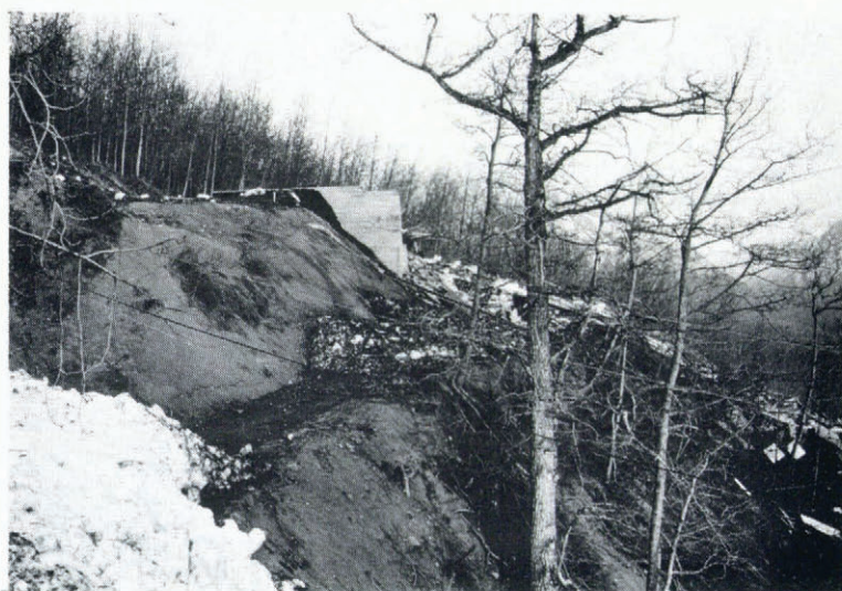
Fig. 14. The foundation remnants of a > $65 000 house that was completely destroyed by a wet snow avalanche during April 1979, Eagle River area, Municipality of Anchorage (photograph by J. Hackett).
