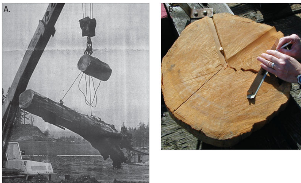
Figure 3. Powerhouse tree. (A) Photocopied photograph from February 17, 1978, issue of the Skamania County Pioneer of tree being extracted during the 1978 excavation of the second Bonneville Dam powerhouse; courtesy of Tim Collins, Bencor Corp., personal communication to Pringle, 1998. (B) Sampling the round conserved at Willamette Locks Museum; photograph by Patrick Pringle.
