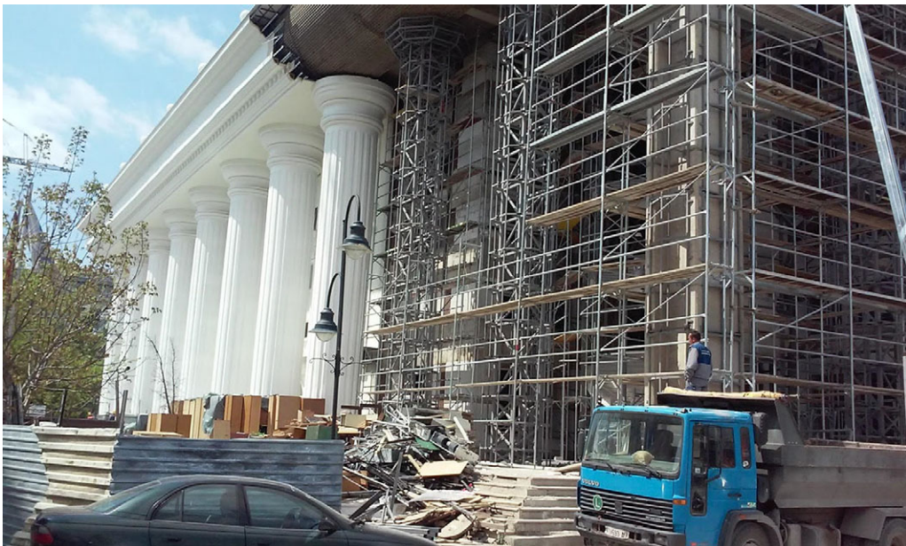
Figure 3. Putting on a new neoclassical façade, covering the modern architecture. Photo by the author.
