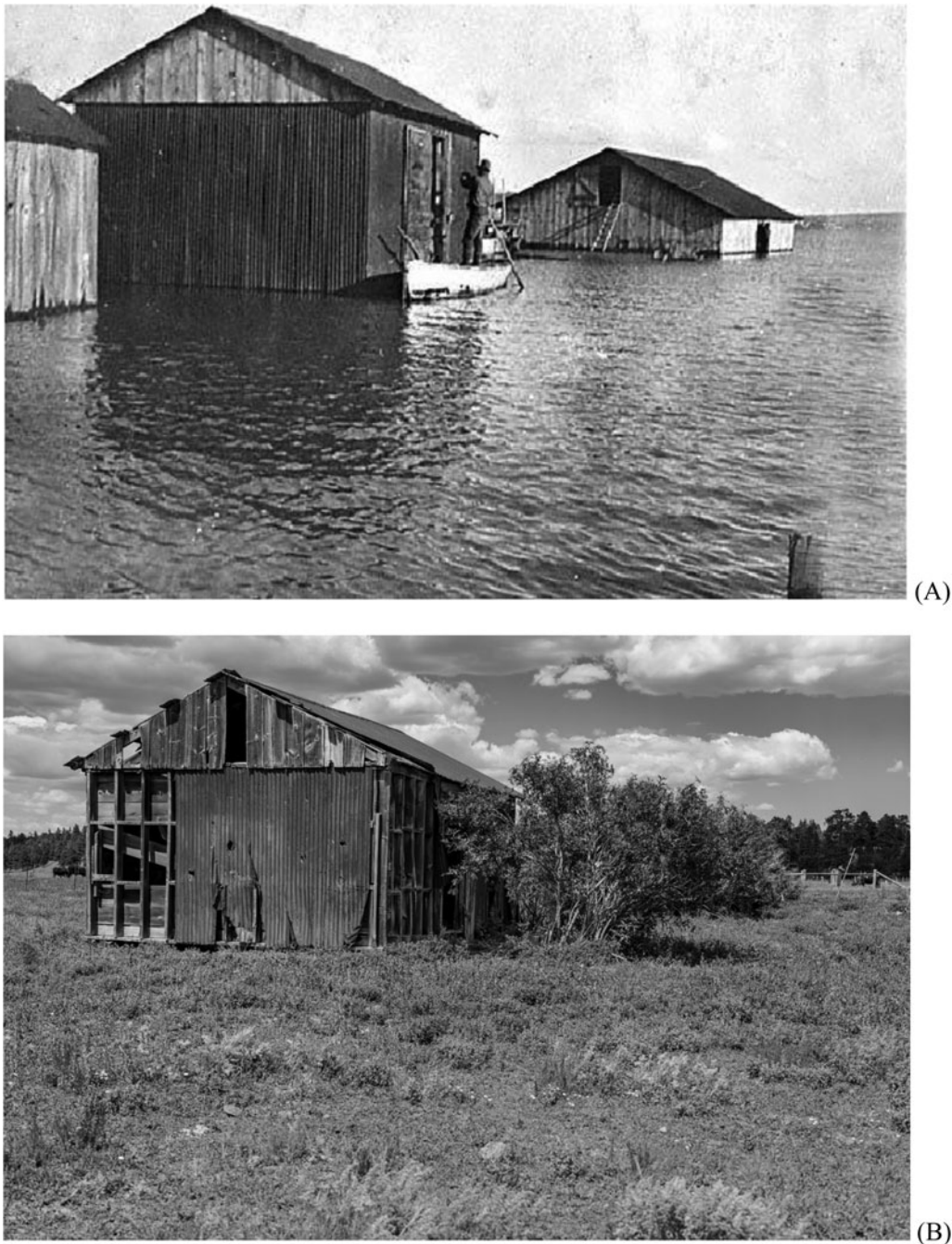
Figure 3. Grass Tank berm, 1920. (A) North-facing photograph of flooded milking barn and two outbuildings (constructed on the berm) when the lake was at its historic high level, inferred water level is 7.9 m; (B) similar scene in 2018, other buildings have collapsed. Courtesy of Cline Library Special Collections, Northern Arizona University.
