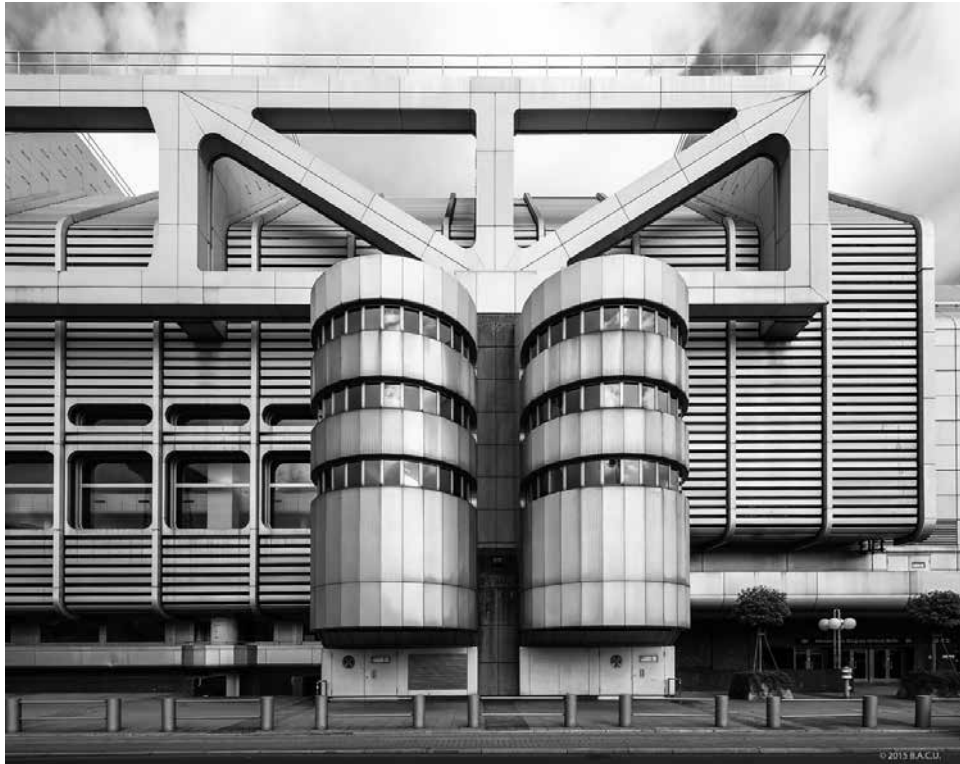
4 International Congress Centre Berlin. Façade detail with stair towers.
