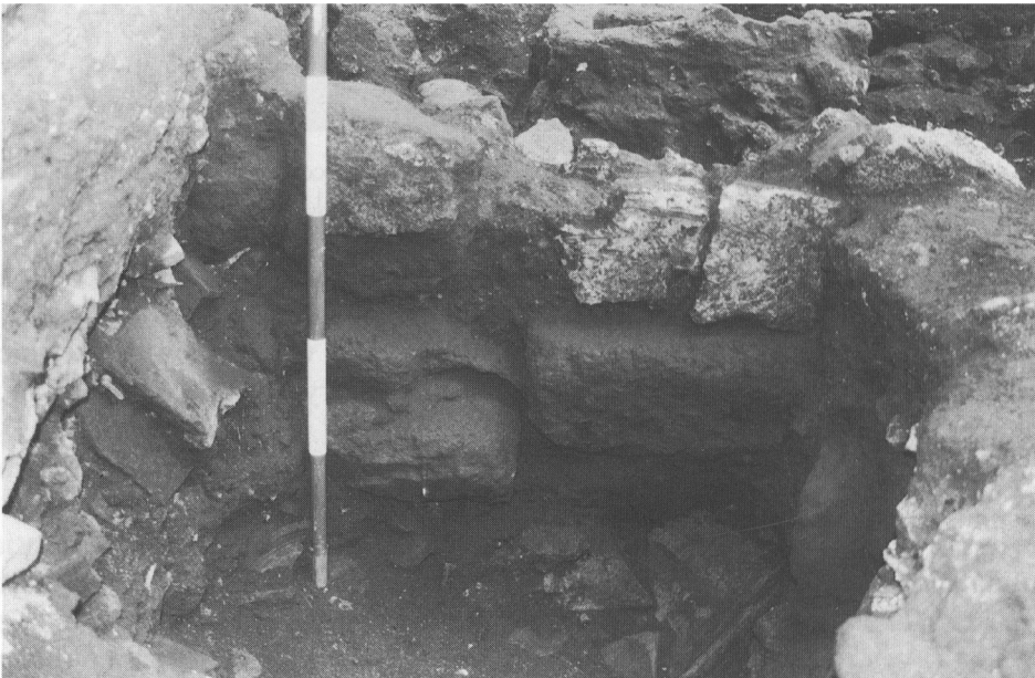
FIG. 13. House 11.5: view of east elevation of early wall 539/605 from the later pit 487. Pappamonte beneath Sarno blocks.
