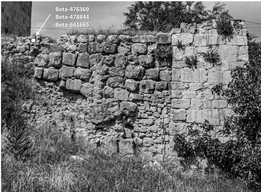
Figure 6 Arubah watermill WJ-02: Southern elevation and sample locations (2 m pole).
