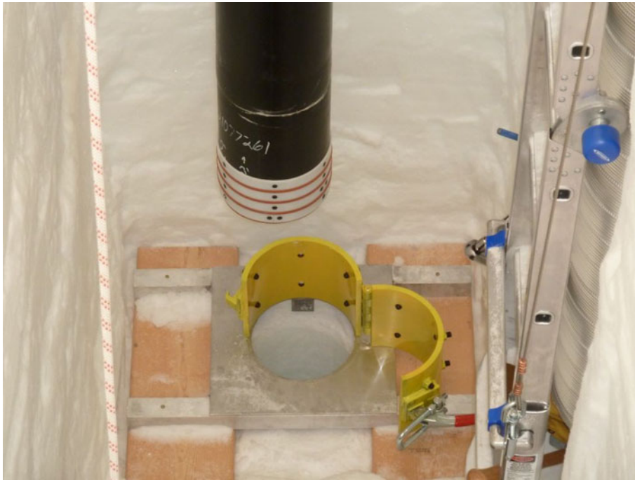
Fig. 11. Casing shoe with sealing O-rings (orange bands) attached to the first section of casing.
