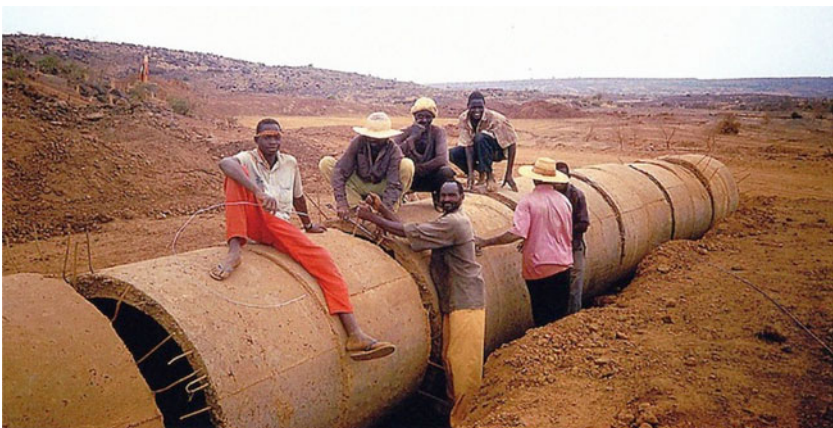
Figure 7. Spillway assemblage.
