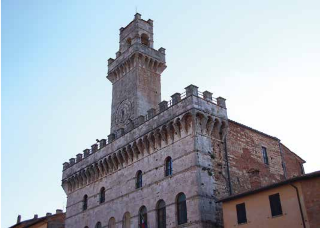
Fig. 5. Montepulciano, Palazzo Comunale, upper portion, view from the northeast, photograph of 2016 by the author
