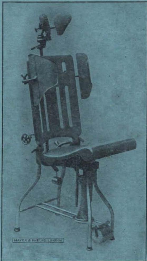
The head rest can be moved in all directions, and locked with one lever in an absolutely rigid position. One pad placed on the left side of the head, the other behind the occiput, leaves the right side of the head free for operative work, and vice versa, a forehead band holding the head immovable.
