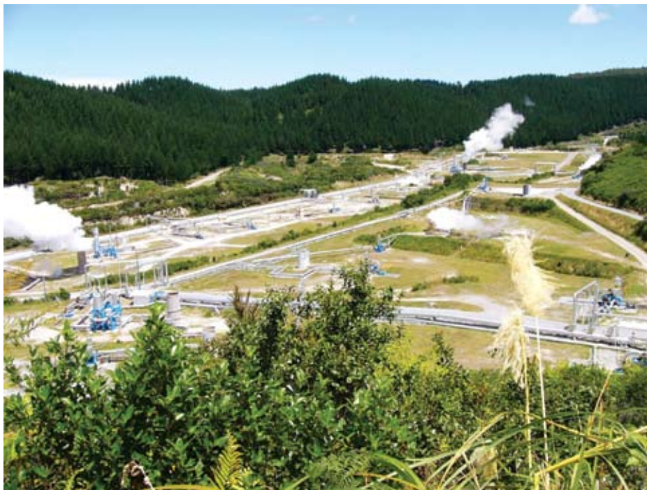
Figure 3. Geothermal field (180 MW) established in 1956 at Wairakei, New Zealand, with bores collecting high-pressure steam for delivery in steel pipes to the power plant located 1 km away adjacent to the Waikato river used to provide cooling water.
