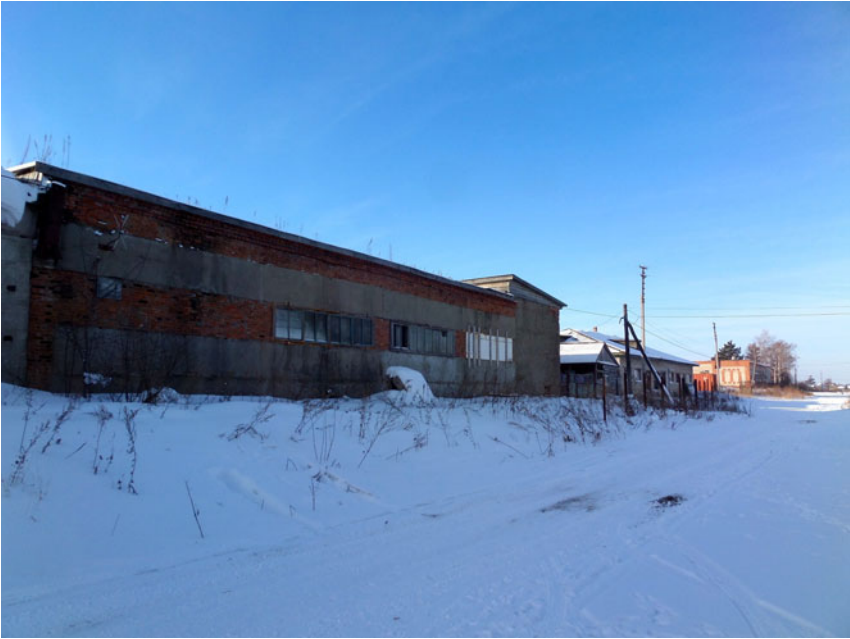
Figure 6. Former Novyi Put' fishing collective, Daerga. Source: Photo by author.
