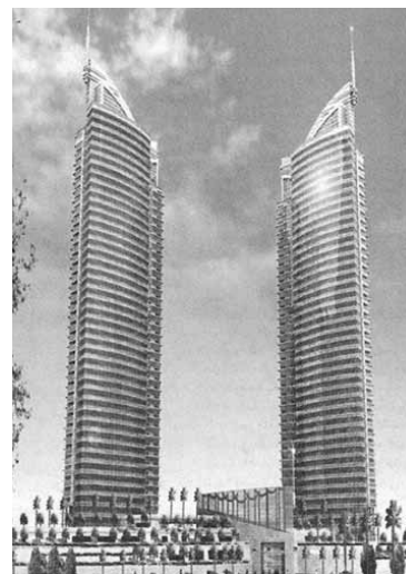
Image of the Jordan Gate project, currently under construction in Amman
