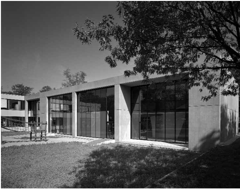
Two projects by Karle / Buxbaum: Protestant Regional Administration building in Gernsheim (top), won through a competition, and the extension to Käthe-Kollwitz Primary School in Darmstadt, a direct commission
