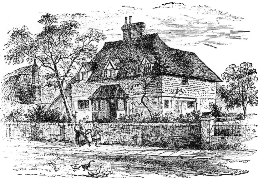
Figure 3. Cranleigh Village Hospital, original building.
