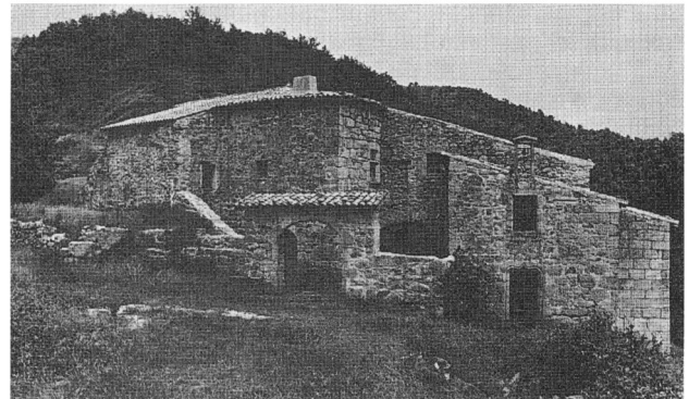
FIG. 1. The main buildings of St Sorny, with the entrance to the disused chapel on the right. The roofs are everywhere sound and professionally supervised at least twice-yearly, and there is rubber-mattress sleeping provision on wooden floors for about 30 boy-scouts, girlguides, or schoolchildren.
