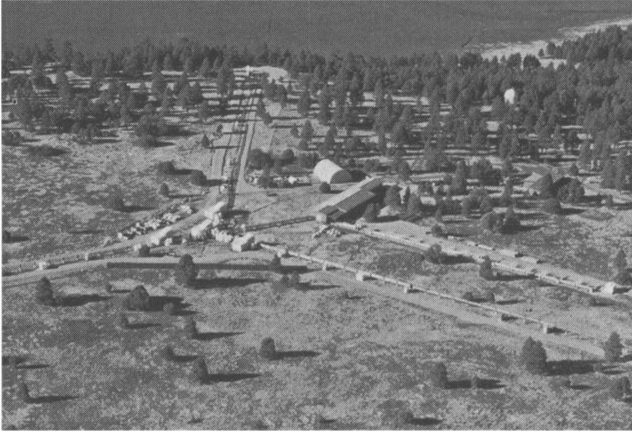
Figure 1. An aerial view of the NPOI showing the array as viewed from the northeast. The road surrounding the array can be seen along with parts of the north (right) west (center) and east (left) arms of the imaging array (station piers and vacuum feed lines visible). The astrometric siderostat shelters are the white structures at the array center. The beam-combining laboratory is the long structure to the right of the array center, with the 'long' delay line vacuum tanks (under construction) extending towards the north. The interferometer control building appears at the far right-center.
