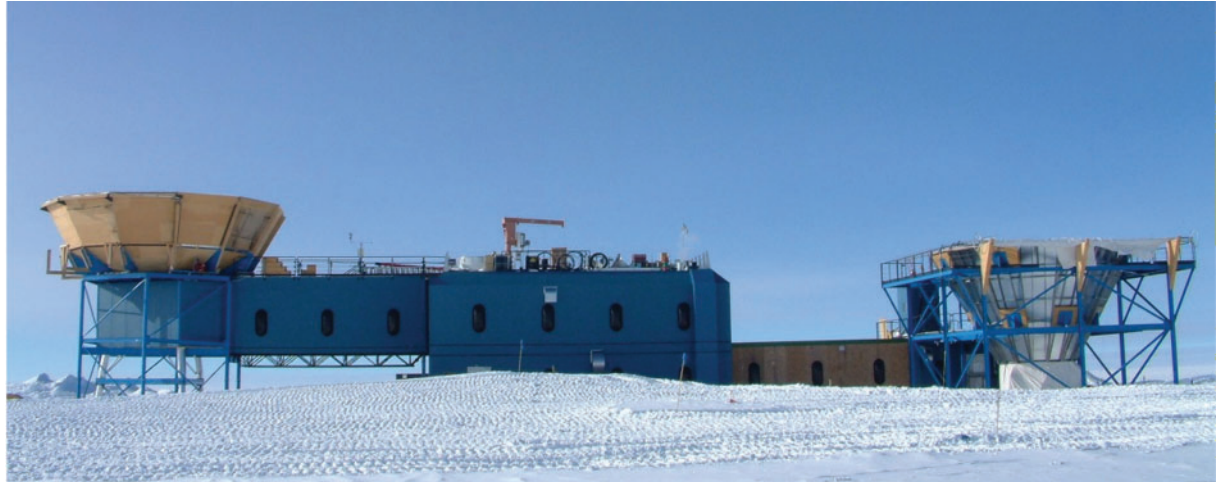
Figure 4 The Martin A. Pomerantz Observatory (MAPO). The 60-cm SPIREX infrared telescope was originally hosted on the tower on the left. In 2000 the DASI CMBR telescope was installed in its place. To the right is the Viper telescope, a 2.1-m off-axis telescope which hosted the ACBAR and SPARO instruments, used for CMBR studies and for mapping polarisation at submillimetre wavelengths, respectively. Image provided by the Office of Polar Programs, National Science Foundation.
