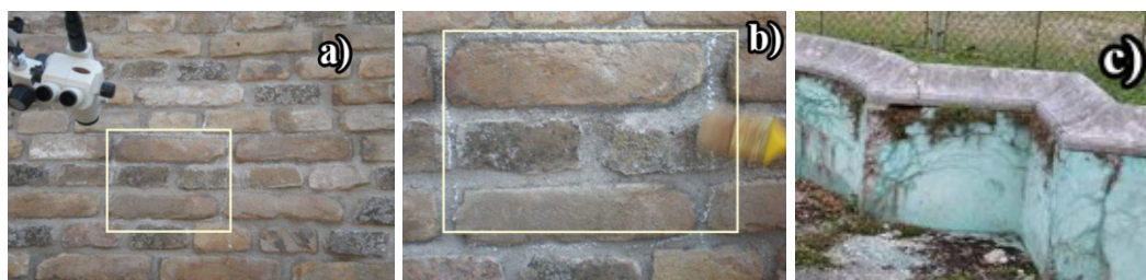
Figure 1. a) Tunnel of the Petrovaradin Fortress before the suspension application; b) Tunnel of the Petrovaradin Fortress immediately after the suspension application; c) Dornava Manor fountain before application
