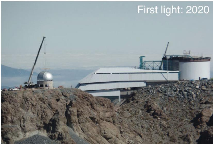
**Figure 2.** The figure shows a photograph of the LSST summit at the time of this Symposium (September 2017). First light for LSST is expected in early 2020 with a 144 Mpix engineering camera, and with the full 3.2 Gpix camera in late 2020. The small dome on the left is an auxiliary telescope that will be used for photometric calibration. For more photographs, see <https://www.lsst.org/gallery/image-gallery>. Credit: LSST.
