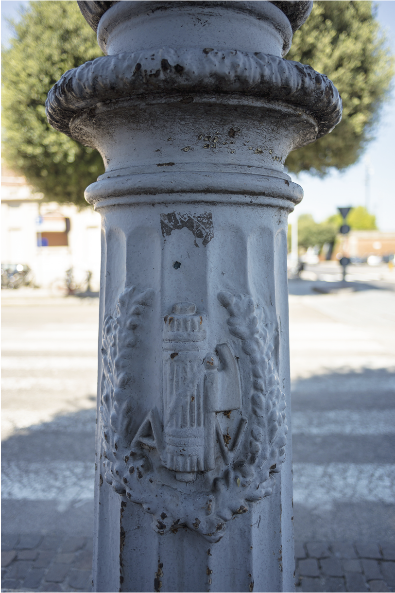
Figure 5. A fasces on a streetlight in Mussolini Avenue. Photo courtesy of Giorgio Casa.
